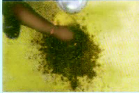
Mix the sand & soil and wet with little water
